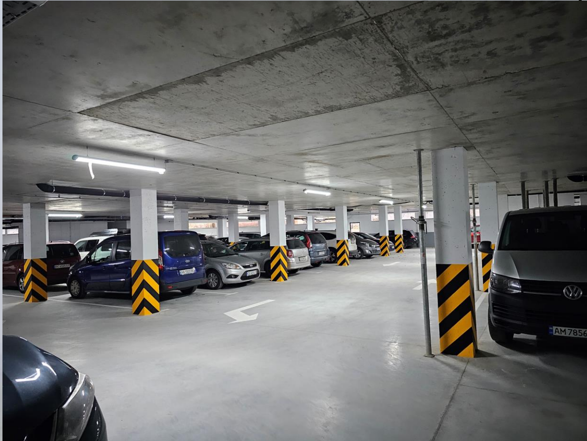
Underground parking at UBTS
