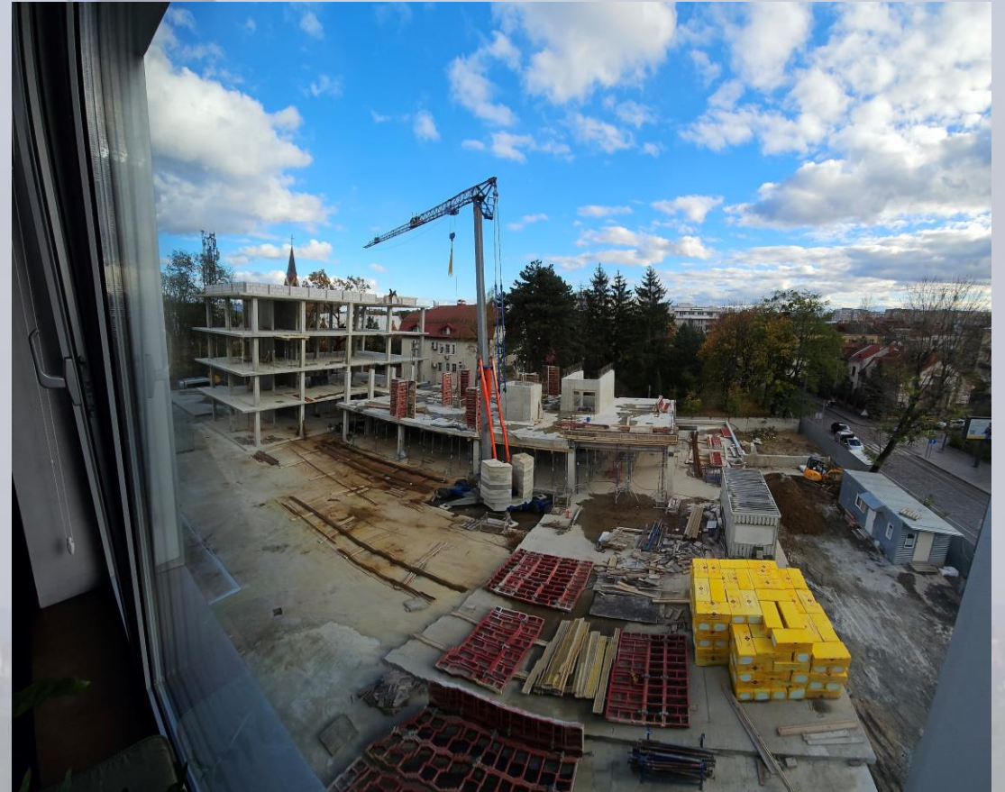
New dormitory construction at UBTS
